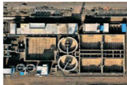
Common Effluent Treatment Plant 20 MLD Commissioned, expandable up to 60 MLD
