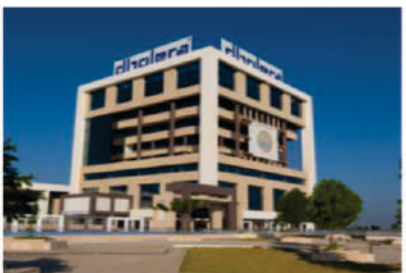
ABCD Building Administrative Building with City Integrated Operation Center
