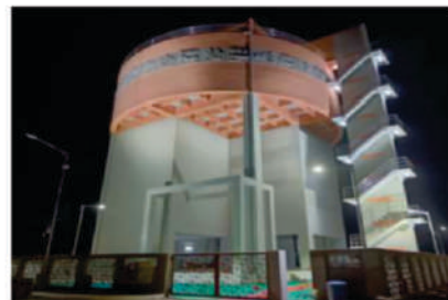
Water Supply & Storage Infrastructure 2 Master Balancing Reservoirs and 9 Elevated Service Reservoirs
