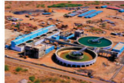
Water Treatment Plant 50 MLD Commissioned, expandable up to 150 MLD
